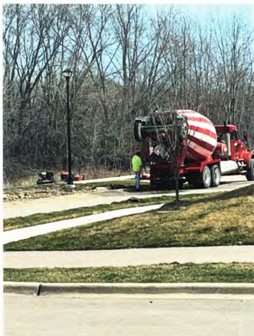
Ozynga Concrete washing their truck shoot directly into the curbside inlet. This is adjacent to what the SWPPP listed as a protected wetland
